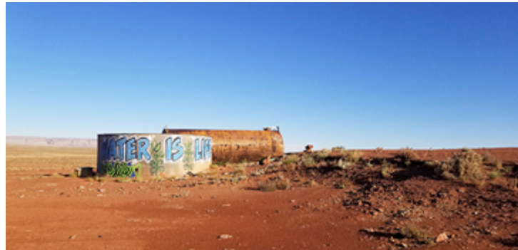
Water Tank located on the Navajo Nation that depicts the arid landscape of the region. Photo Credit: Carlee McClellan, NNDWR partner.
